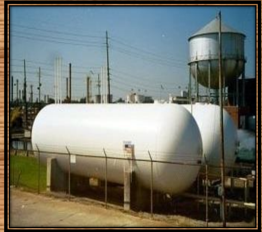
Chlorine Gas Storage Cylinder
