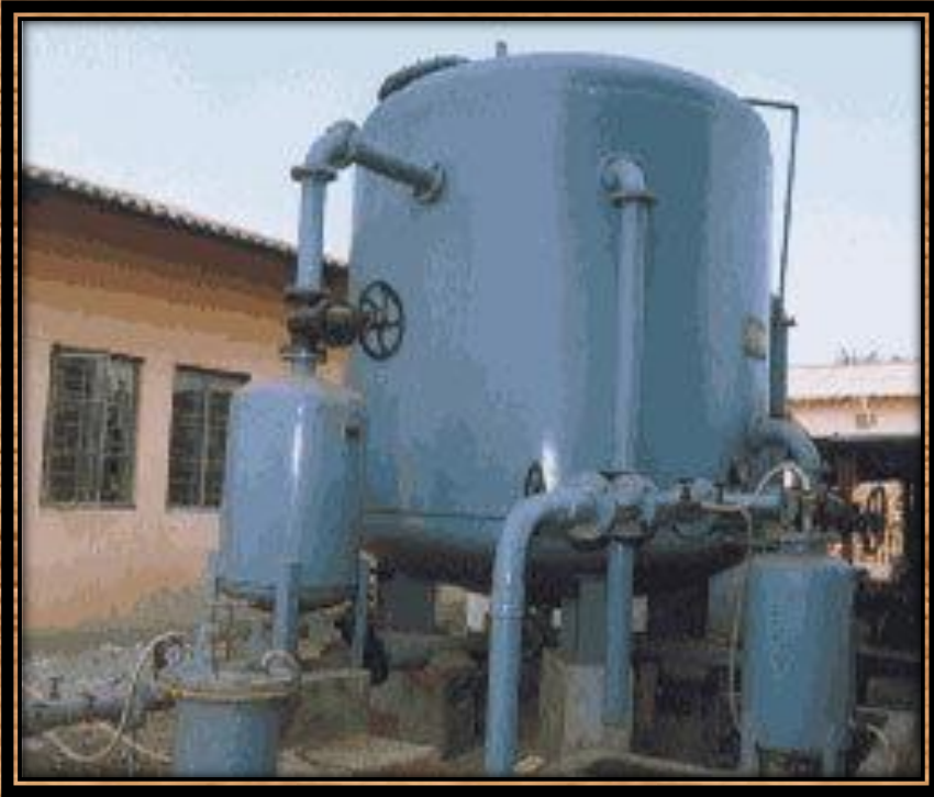
Chlorinator with Separator and Agitator
